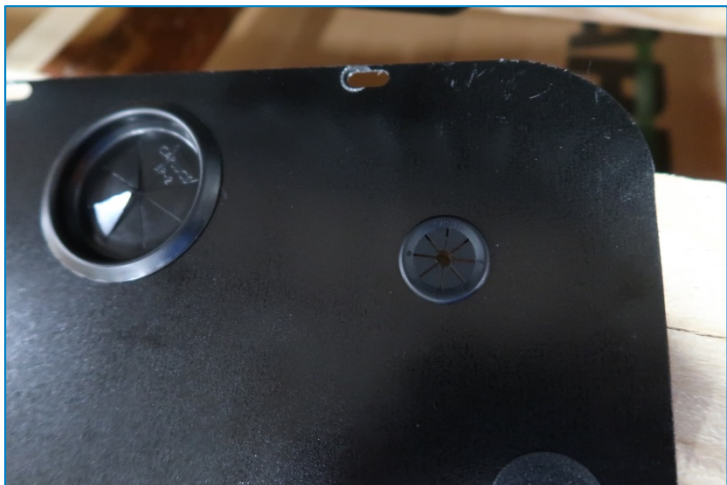
Low voltage wiring entrance grommet installed
