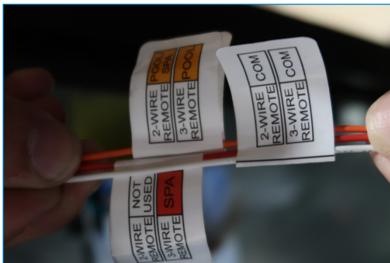
Low voltage wire labels
