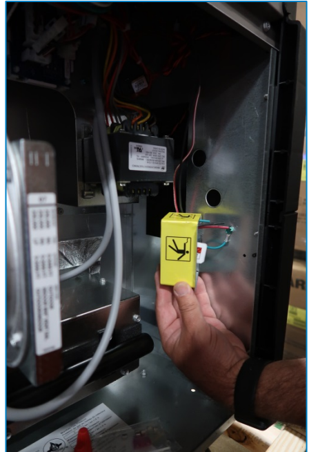
High Voltage Junction Box relocated to right side
