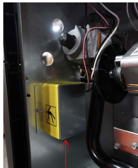
High Voltage Junction Box
